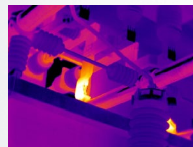
Infrared thermal image
